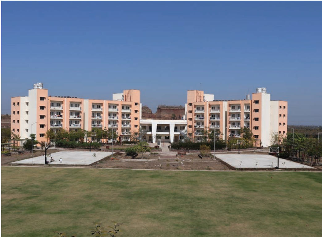
Hostels and Mess Block: NID MP campus
