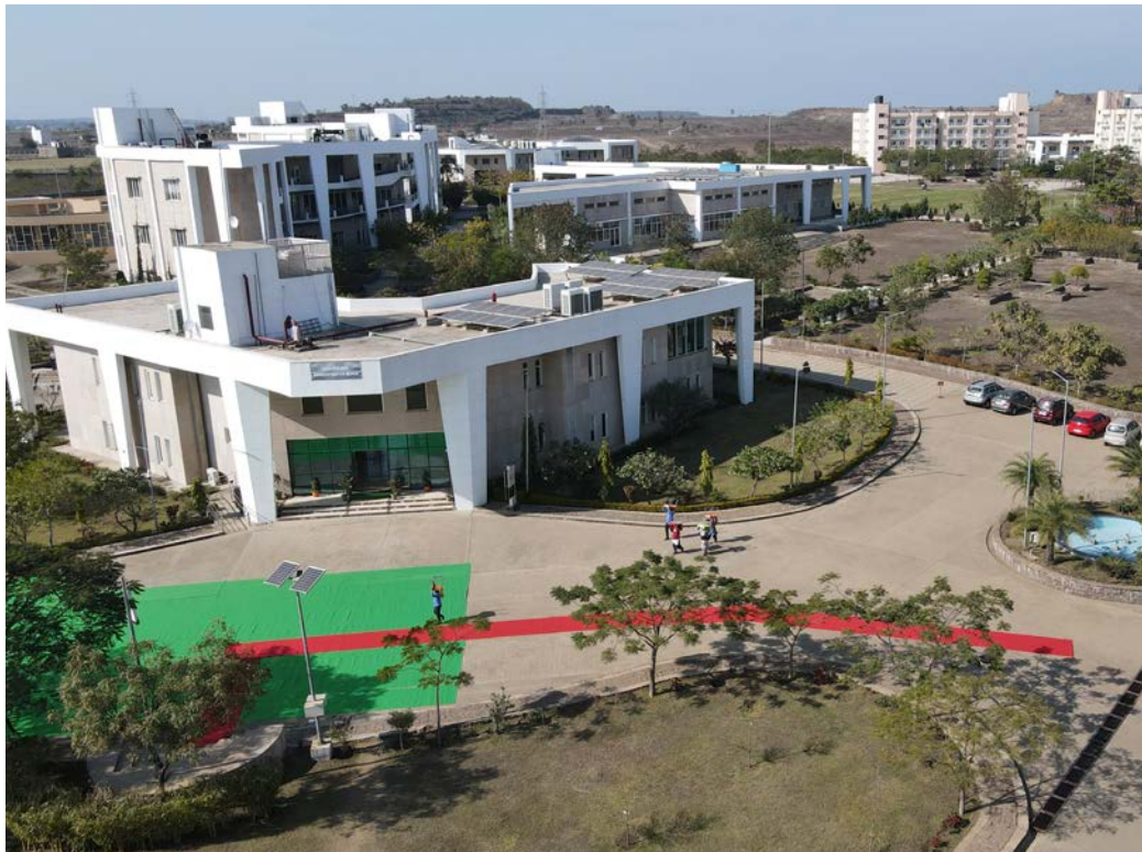
Administrative Block: NID MP campus
